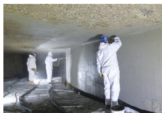
MC News Potable water tank in Oberwart repaired Page 11
