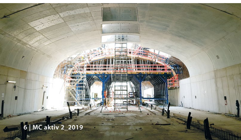
View of the sealed S-Bahn (metro) station.
