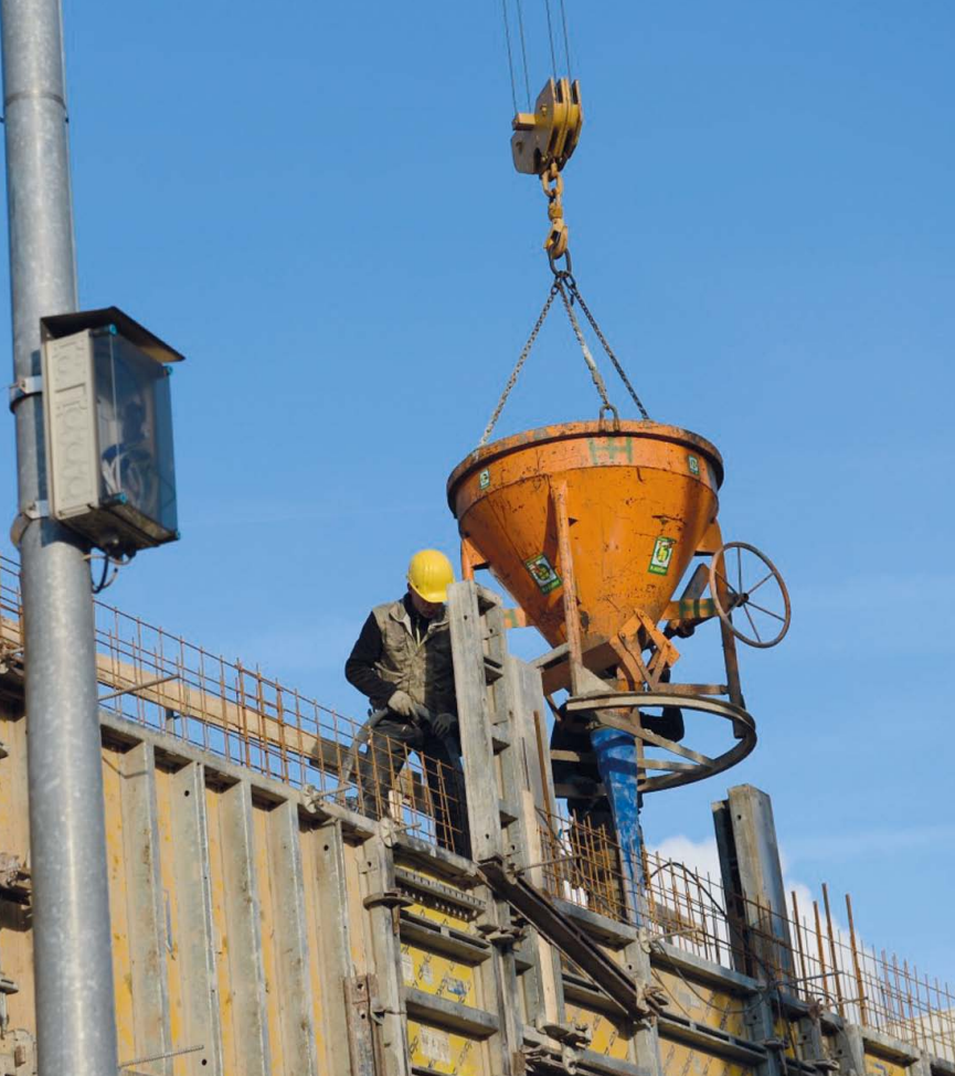
Concrete work in the construction of new facilities at MC-Bauchemie, Bottrop, in 2016.
