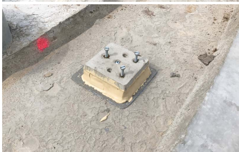
MC-AnchorSolid E280 was used, among other things, for anchoring and bonding the bearing blocks* for the first tower ring on the foundation of the wind turbine masts.
