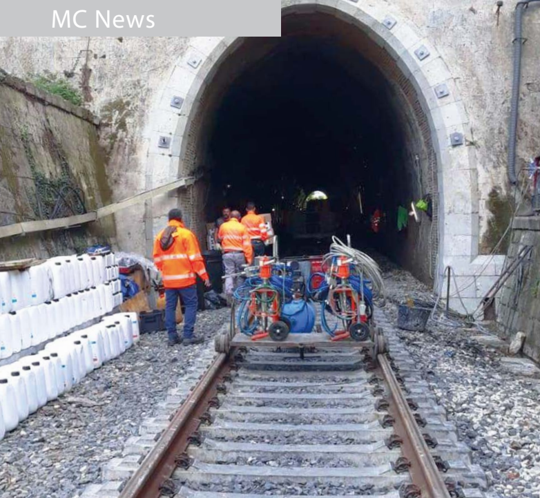
The tunnel was sealed with a curtain injection using the elastomeric hydro-structural resin MC-Injekt GL-95 TR.
